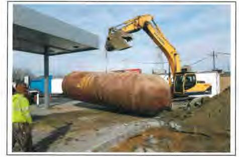
**DESCRIPTION:** View of UST removed and preparing to be cut/cleaned
