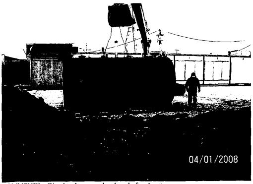
COMMENTS: Diesel tank removed and ready for cleaning.
